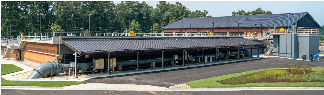
James E. Quarles Plant 1 Replacement
