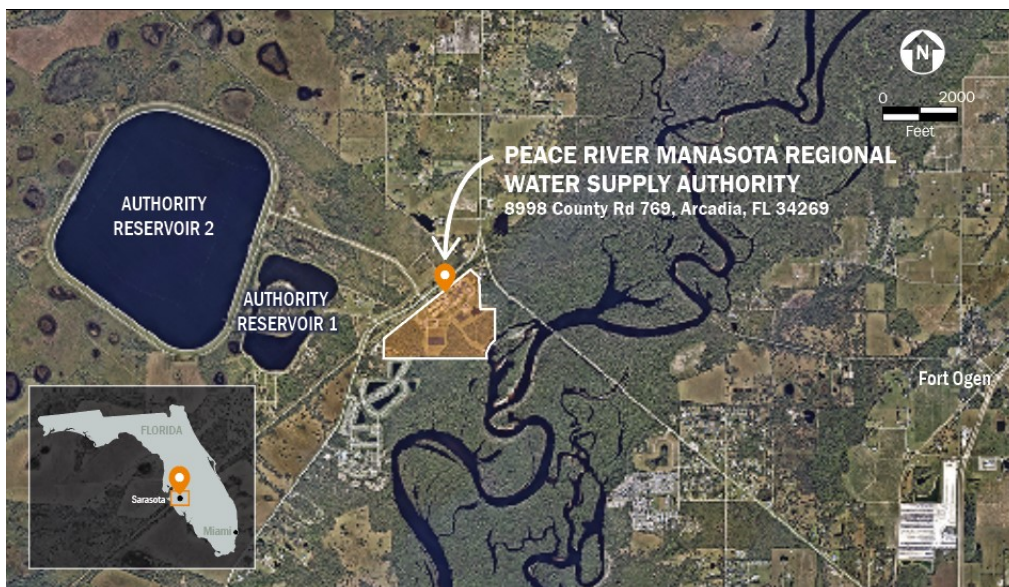
Figure 2-1. Aerial View of Peace River Facility
