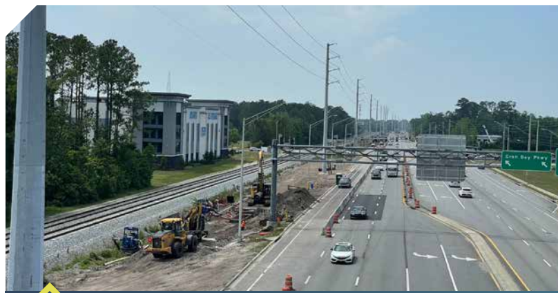
WORKING WITHIN AN EXISTING RAILROAD & FDOT RIGHT-OF-WAY
