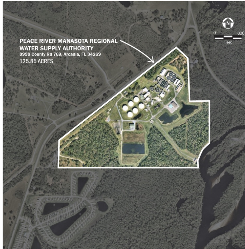
Figure 2-2. Aerial of Peace River Facility Water Treatment Plant
