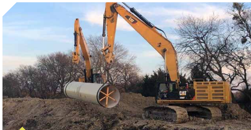
84" DIAMETER C200 STEEL PIPE BEING INSTALLED OVER A COMBINED 56 MILES
