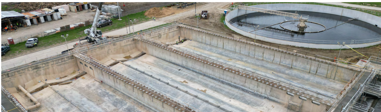
South Mesquite Creek Regional WWTP
