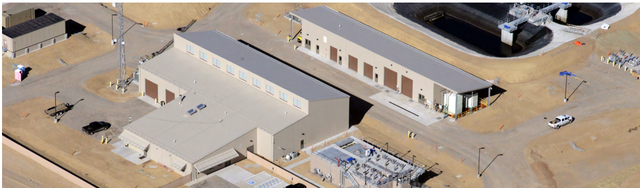
Cutter Lateral Reach 21 Water Treatment Plant
