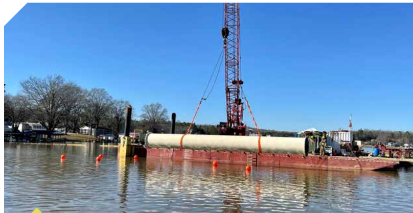
MARINE CREWS INSTALLING 54" COATED STEEL PIPE
