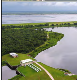
Pump Station from Res No. 1
