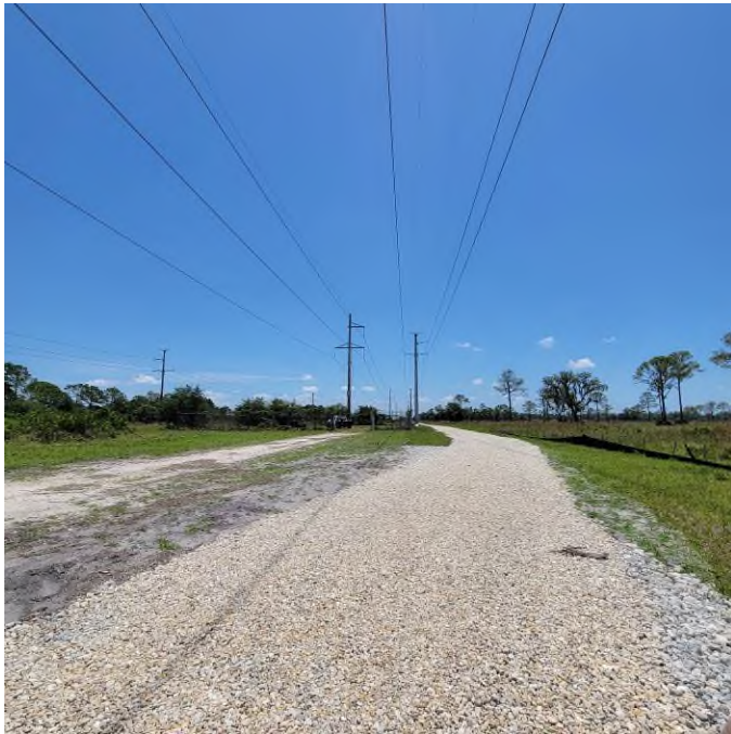
View of Gravel Road Running Along FP&L Easement)
