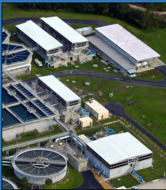
The Filter Covers at the Peace River Facility
