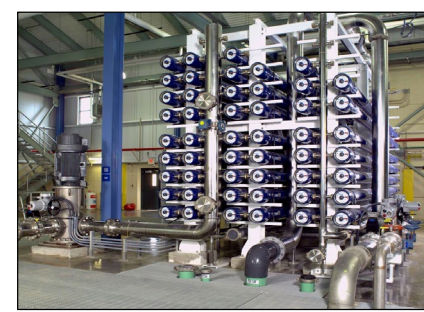
Typical RO systems have arrays or modules of vertically stacked pressure vessels, leading to a compact overall site footprint
