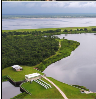
Pump Station from Res No. 1
