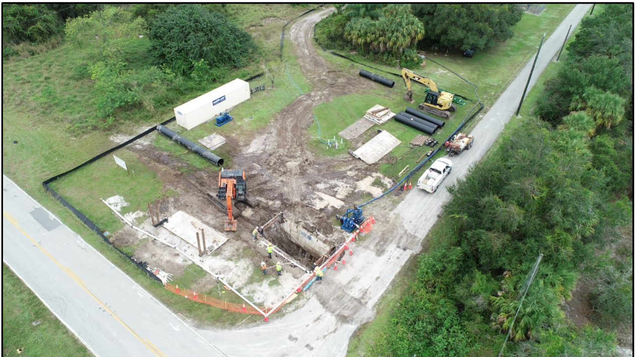
Jack and Bore Preparation at Shell Creek Reservoir, Dam Road – South Side of Shell Creek Nov. 2019
