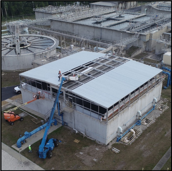
Plant 1 - Installation of Roof Pans
