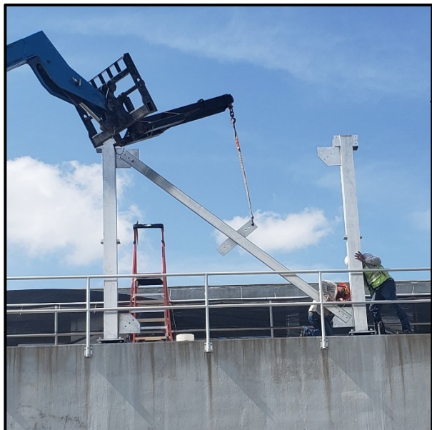
Plant 1 - Vertical Structural Members Installation
