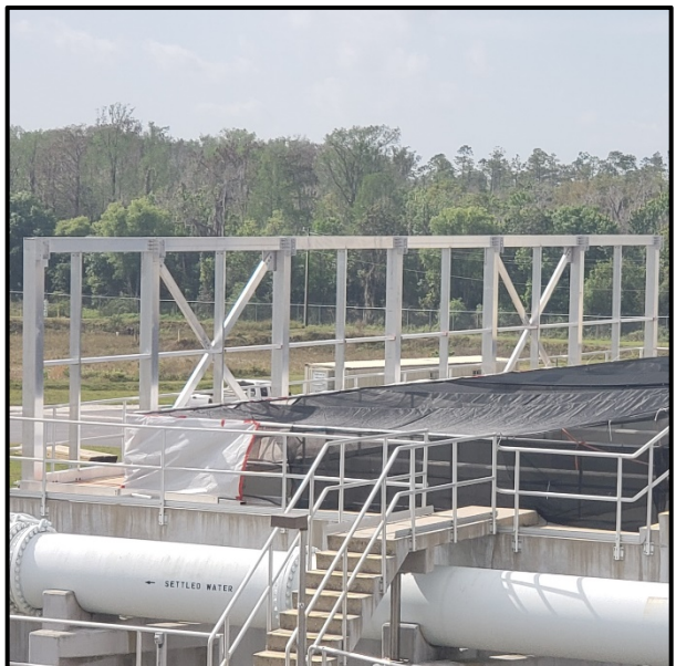
Plant 1 - Vertical Structural Wall Completed
