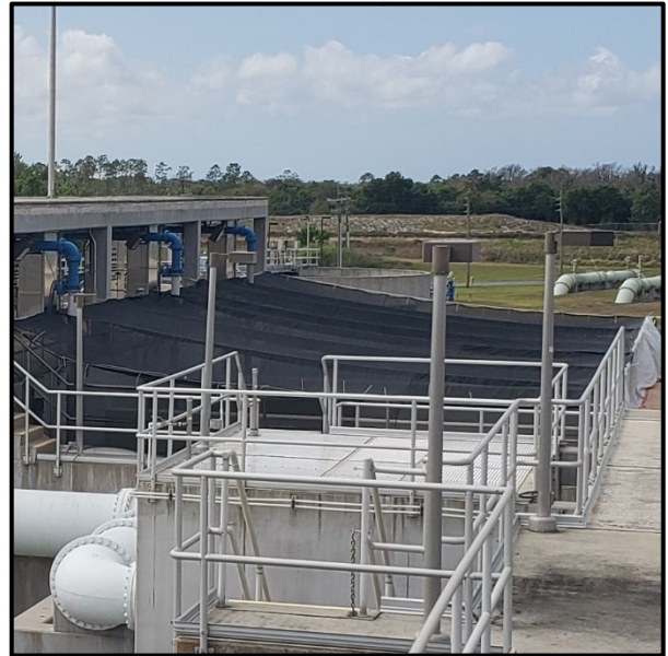
Temporary Protective Cloth Over Filter Basin
