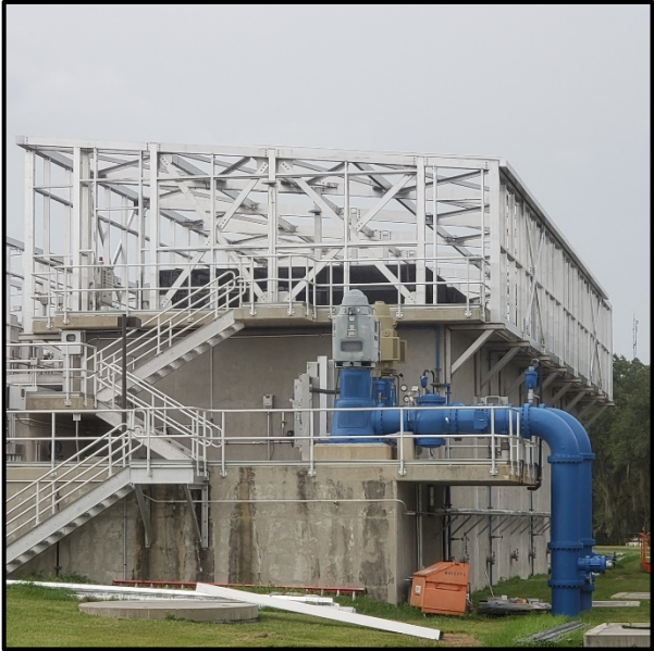
Plant 4 – Completed Structural Framing
