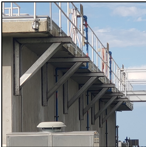
Plant 3 – Outer Wall Column Support Brackets
