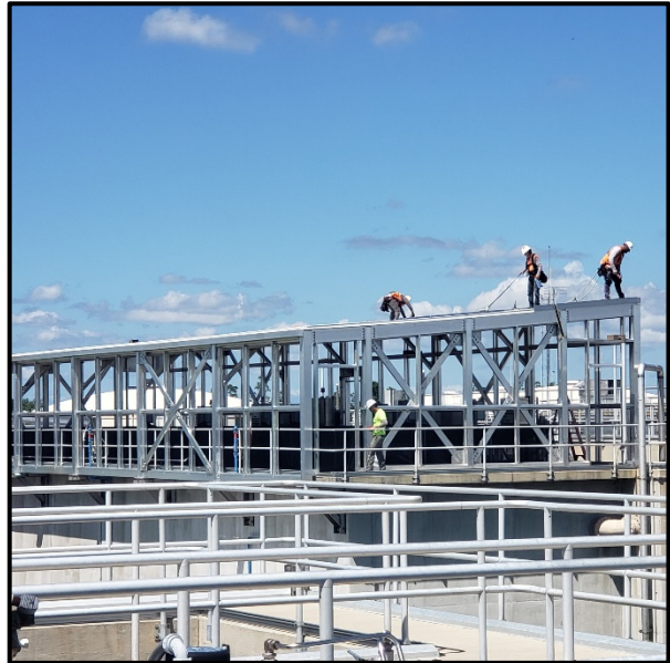
Plant 2 – Installation of Roof Pans
