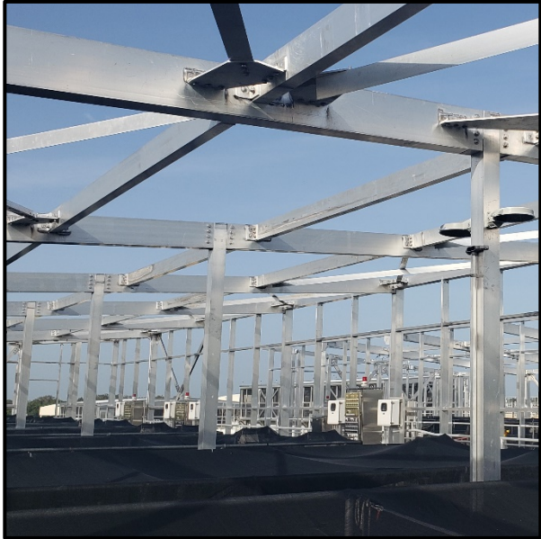
Plant 4 – Temporary Filter Basin Protection
