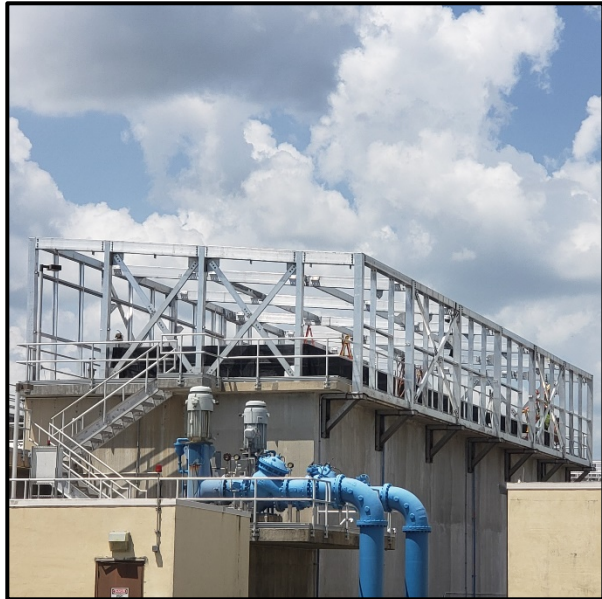
Plant 2 - Completed Structural Framing
