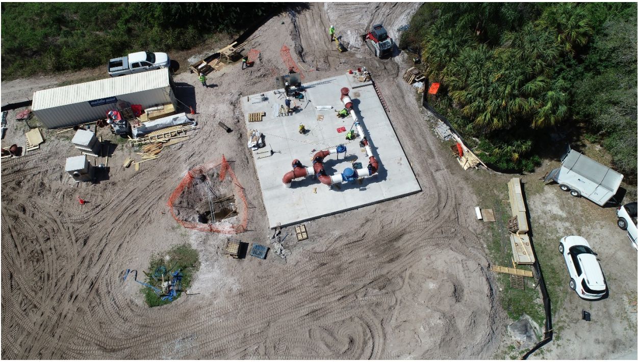
Shell Creek Meter Assembly Construction – March 2020
