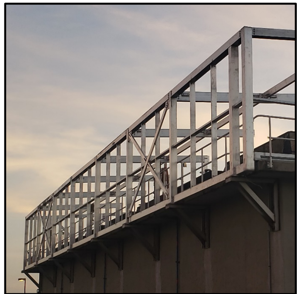
Plant 4 – Completed Outer Wall Framing
