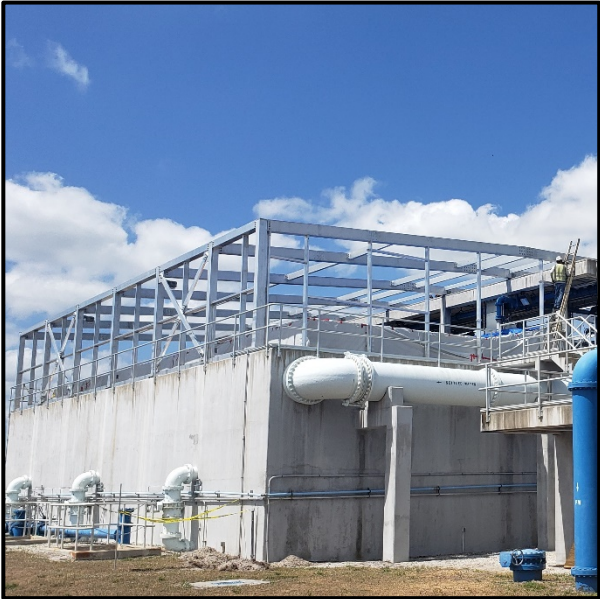
Plant 1 - Completed Structural Framing
