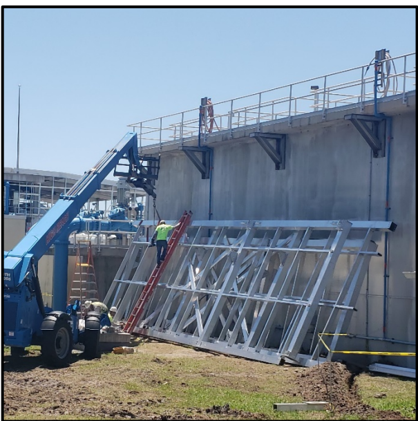
Plant 2 – Installation of Wall Brackets
