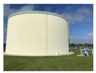
Figure 1-3: 0.5 MG Ground Storage Tank and Recirculation Piping
