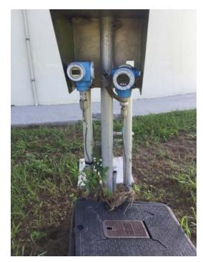
Figure 1-4: Redundant Tank Level Transmitters
