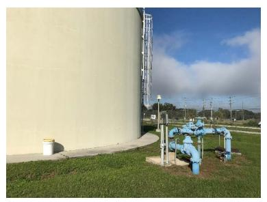
Figure 1-6: Recirculation Pump and Piping
