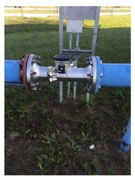
Figure 1-5: Battery Powered Octave Ultrasonic Meter (Influent)
