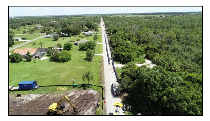
HDPE pipe fused and ready for Pullback on north side of Shell Creek, July 6, 2019
