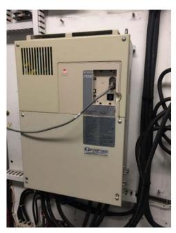
Figure 10: Variable Frequency Drives
