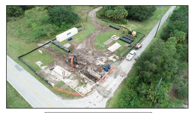
Jack and Bore Preparation at Shell Creek Reservoir, Dam Road – South Side of Shell Creek Nov. 2019
