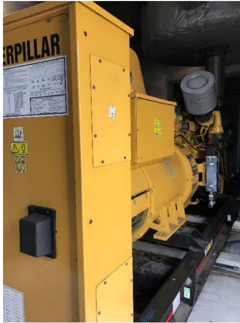
Figure 13: Emergency Generator
