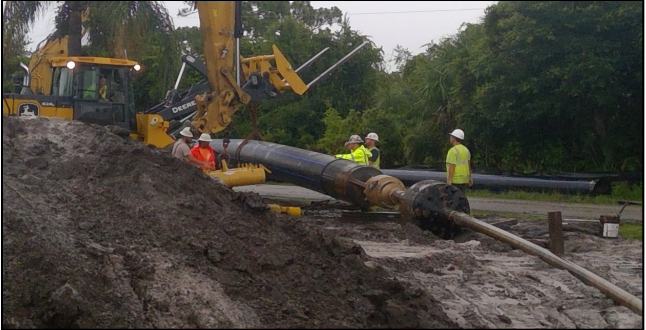
Drill Rod attached to pulling head on HDPE pipe for Pullback - north side of Shell Creek – July 7, 2019
