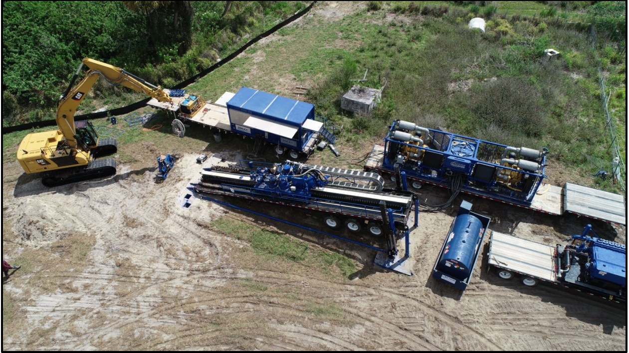
Horizontal Directional Drill Rig
