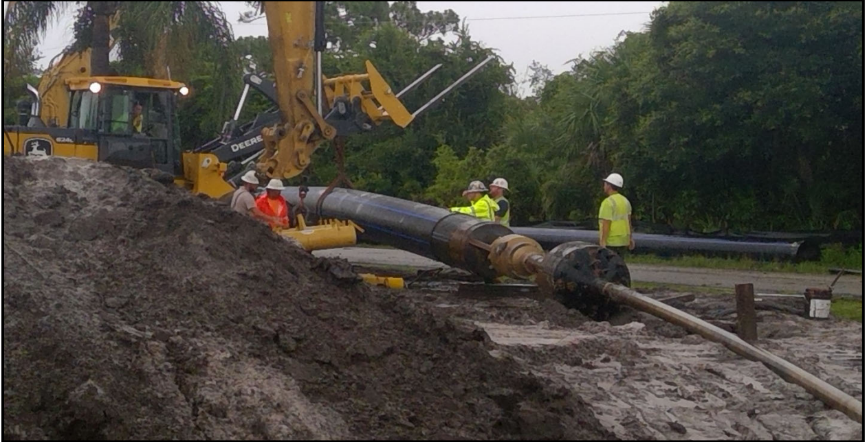
Drill Rod attached to pulling head on HDPE pipe for Pullback - north side of Shell Creek – July 7, 2019
