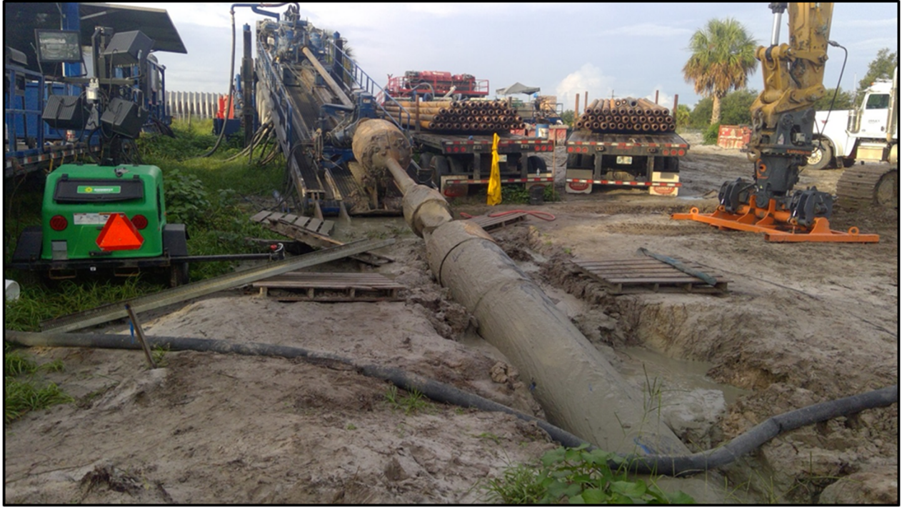
3,500-lf Pullback completed July 8, 2019 South side of Shell Creek
