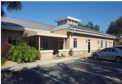
Additional Subject View of the East Elevation and Covered Patio
