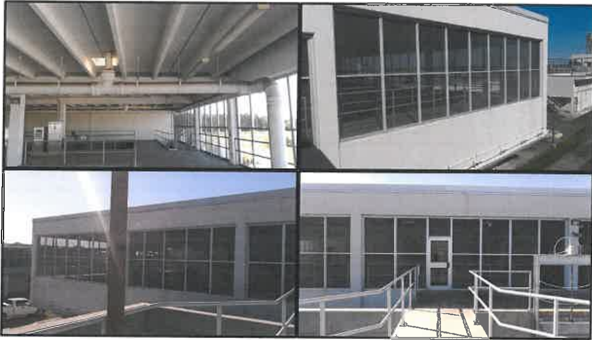
FIGURE 3 – Filter Covers at the Lake Manatee WTP
