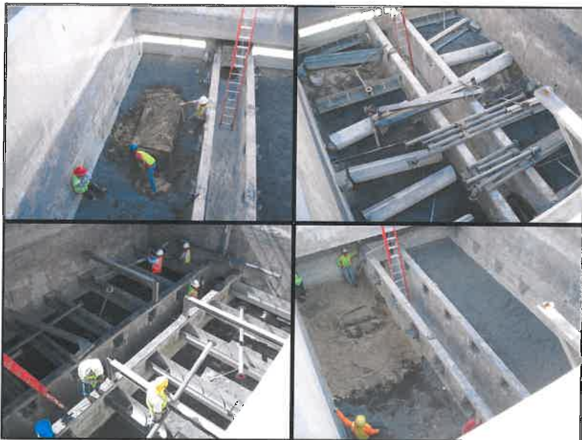
FIGURE 2 – Examples of Work in the Filters during the 1991 Rebuild Project
