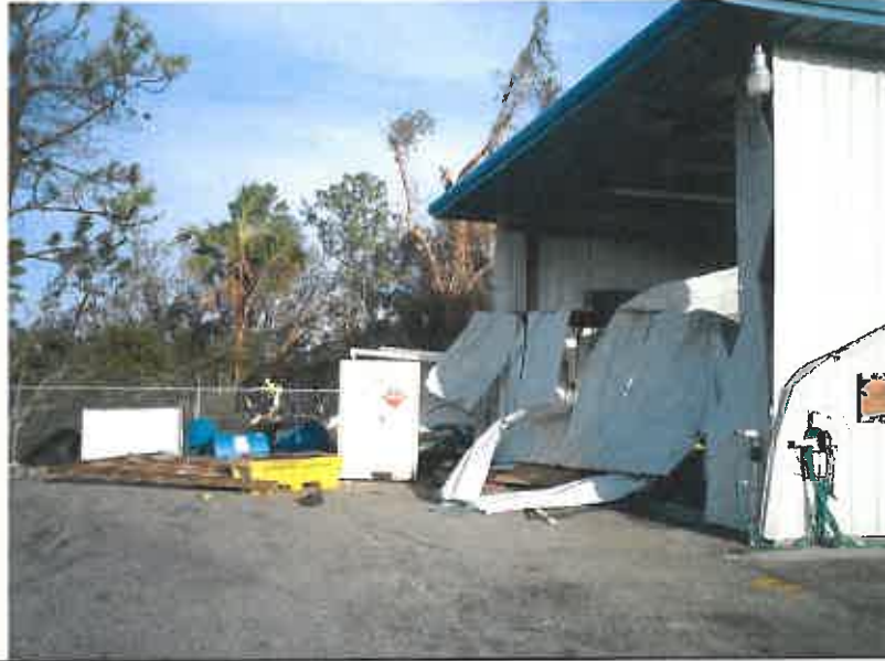
Shell Creek WTP
