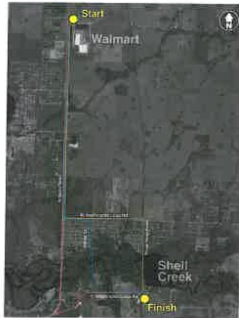
Peace River Manasota Regional Water Supply Authority Regional Phase I Drinking Water Pipeline Project
